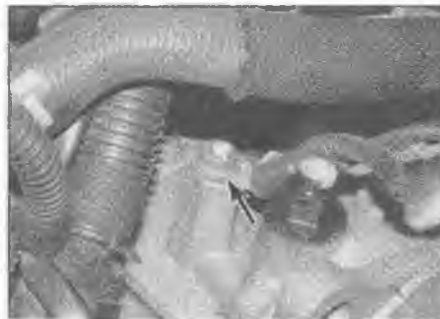
9.3 Engine/transmission earth strap connection (arrowed)
