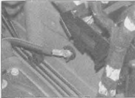
2.20a Earth connection adjacent to the left-hand gearbox mounting ...
