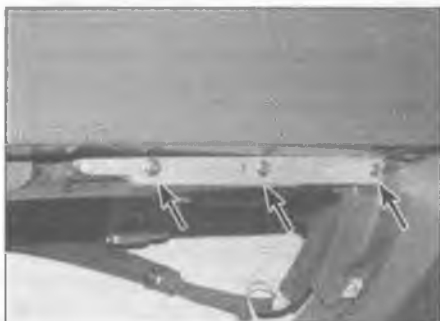
22.9a The fascia covering trim is secured by numerous fasteners along its lower edge (arrowed) . . .
