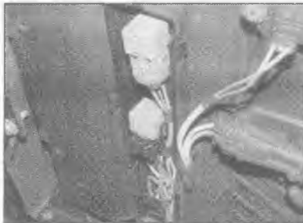
3.8 The cooling fan relays are located in the front panel
