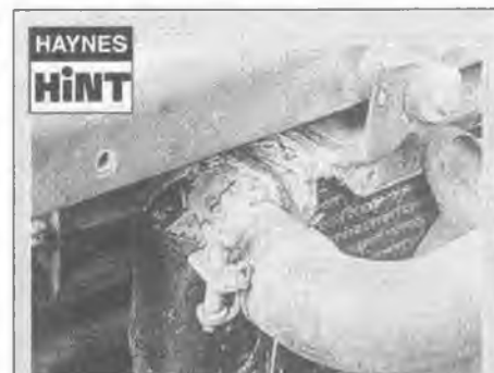
A leak in the cooling system will usually show up as white- or rust-coloured deposits on the area adjoining the leak.
