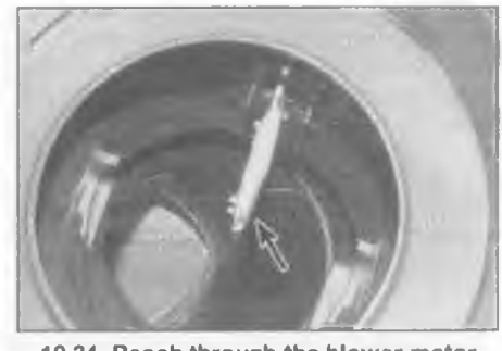
10.34 Reach through the blower motor aperture, and rotate the resistor (arrowed) to remove it
