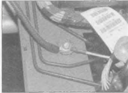
2.20b ... in front of the engine compartment fuse/relay box ...
