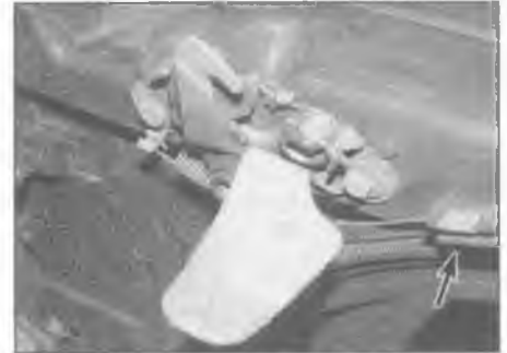
6.6 Undo the bonnet locks bolts, and free the cable from its retaining clips (arrowed)
