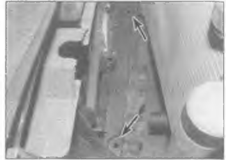
12.14b . . . and lower (arrowed) mountings are correctly fitted
