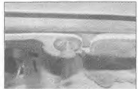
2.39b Lever up the centre pins, remove the rivets, and detach the sound insulation material from the crossmember . . .
