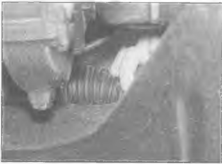
6.2 Check the steering rack gaiters for damage
