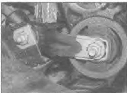
7.18 Undo the nuts and bolts securing the rear engine mounting link
