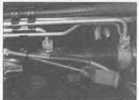
Power steering fluid may leak from the pipe connectors on the steering rack.
