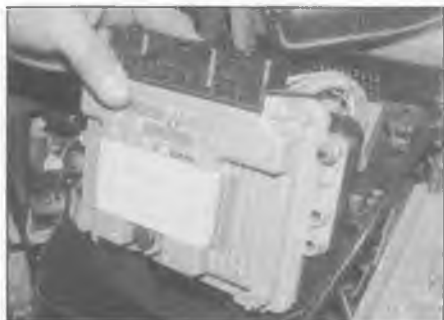
13.7 Lift the ECU from the electrical box
