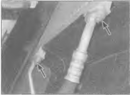
12.12 Undo the nuts (arrowed) securing the refrigerant pipes to the condenser
